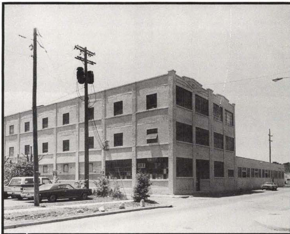
Ideal Motor Car Co. building at 221 W. 10th St., Indianapolis, IN. Original factory of 1911 consisted of the first 2 bays on left side of the 3-story section. Photo #22 taken by Alan Conant, I.H.P.C., 1984.
