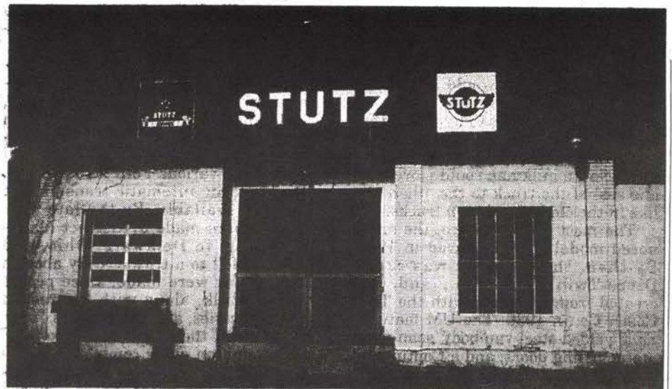
The Stutz fire truck factory as it appeared in 1992.
