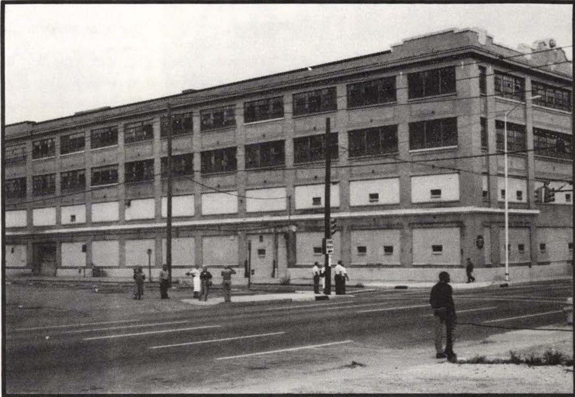
H.C.S. Motor Company Building 1402 North Capitol Avenue
