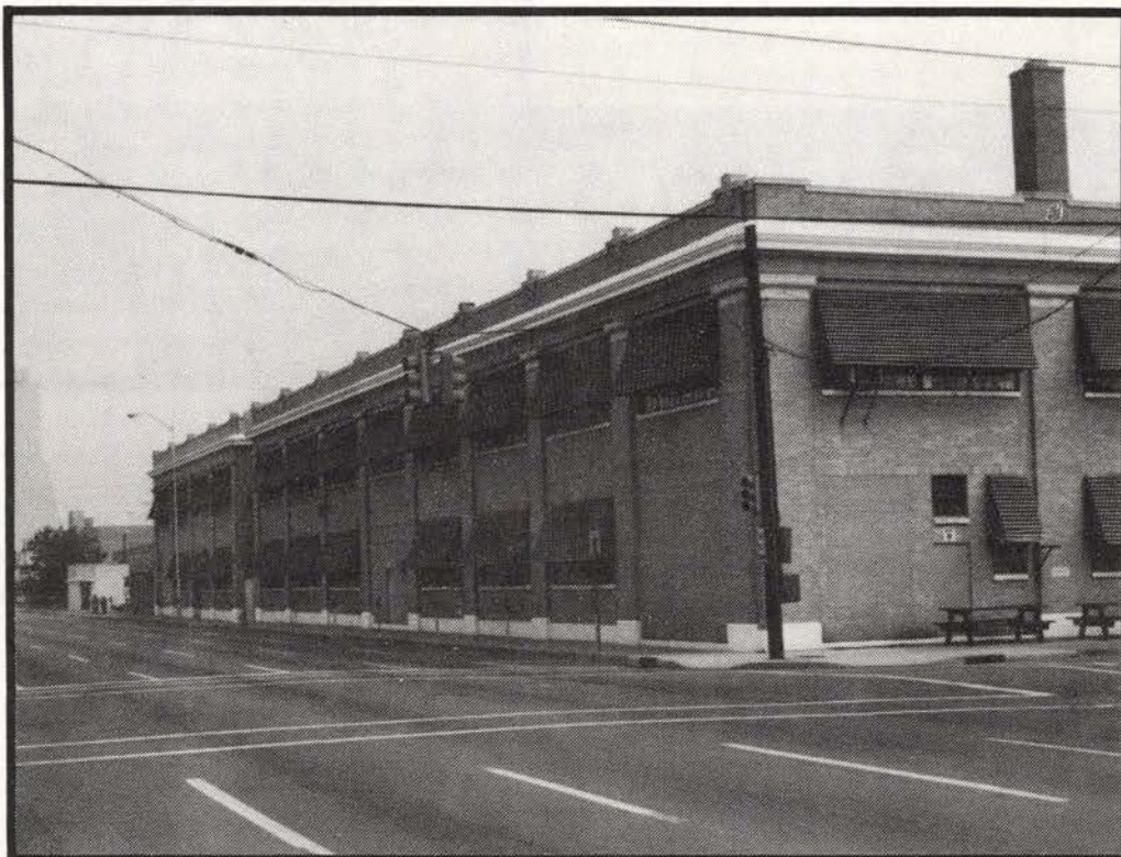
Stutz Fire Engine Company Building 1411 North Capitol Avenue
